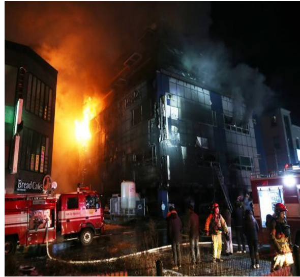
Emergency services at the scene where 29 people died and dozens more were injured in a fire that engulfed a commercial building in the southern city of Jecheon
